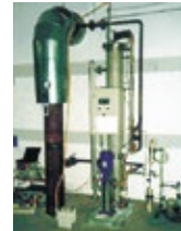
Servitec test facility in a heat transfer station of the energy supply hall
